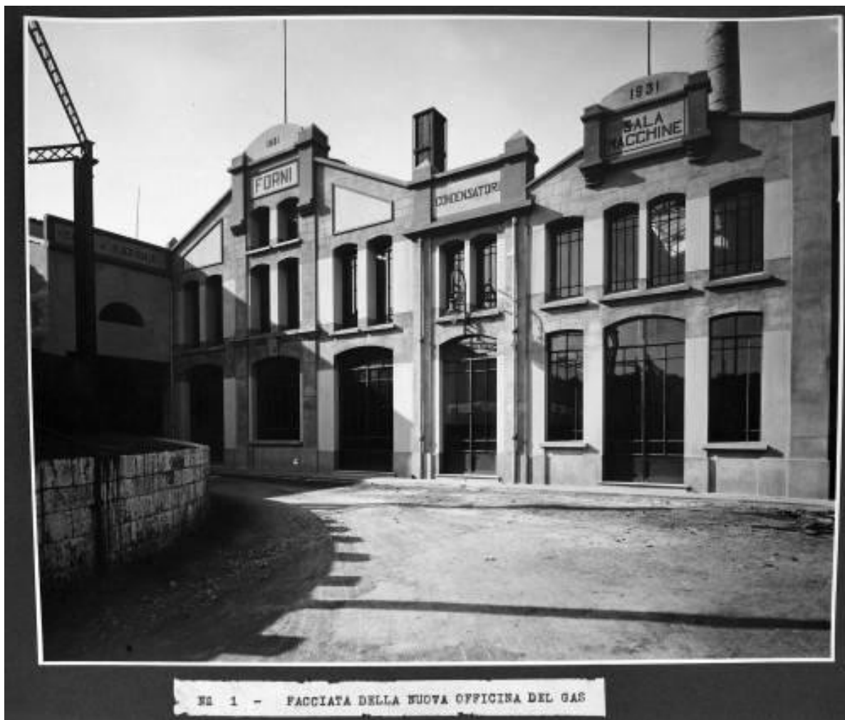
Fig.14. Officina del gas 1931 (AFT)
